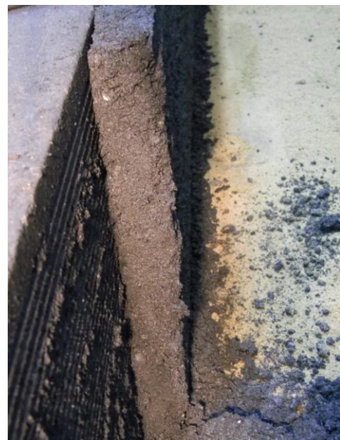
Figure 12. A destructive analysis showed a very homogeneous compaction through the 6 layers, with good layers bonding.
