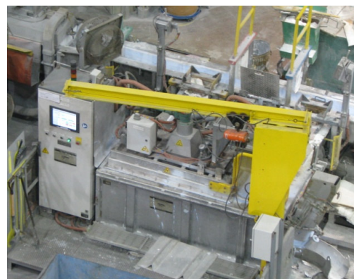
Figure 7. The ACF filter in an industrial environment
